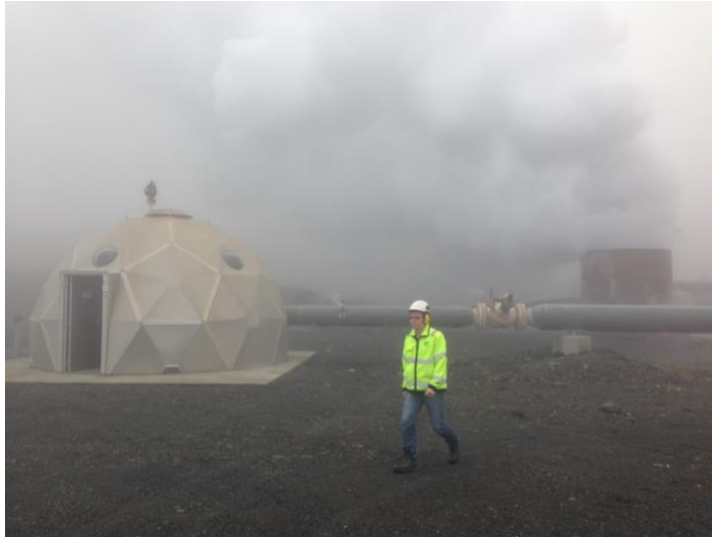
Figure 2: Geologist at geothermal wellhead, Hengill. The wellhead is the igloo like structure to the left of the picture. Following the thick pipe rightwards, there is an additional segment wedged between two pipe sections. The separator is attached here to access fluids. In the background to the right is the silencer. Picture by author.
